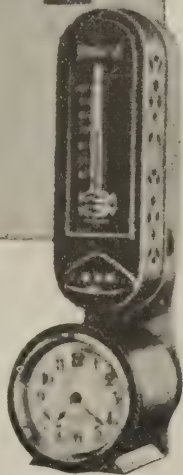
HEATING INSTALLATION UNDER THERMOSTATIC CONTROL. THE THERMOSTAT SHOWN IN THE LIVING ROOM CONTROLS THE MOTOR IN THE CELLAR, WHICH IN TURN OPERATES THE DAMPERS AND DRAFTS
